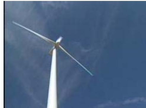
Colorado's new energy economy is getting a boost thanks to Vestas.
